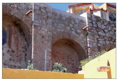
Evidence of damage already inflicted on a centuries old church, due to vibrations from explosions.
