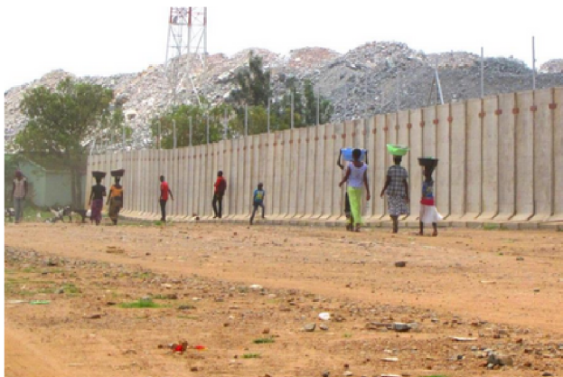
Photo: The above three images show the proximity of public roads and village homes to mine walls and the Nyabirama pit beyond. (Catherine Coumans, MiningWatch Canada, 2018)
