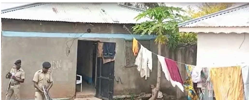
Photo: Police overseeing the bulldozing of houses in Komarera Village. December 2022. (Still from video with MiningWatch)
